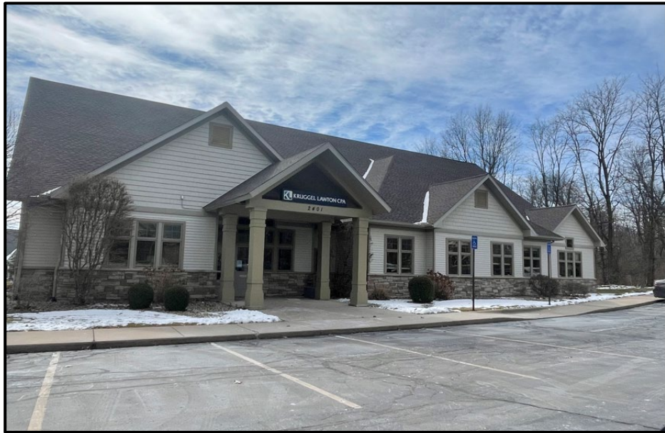
Figure 1. Looking south at entrance of subject building (2401 W Centre Ave).
