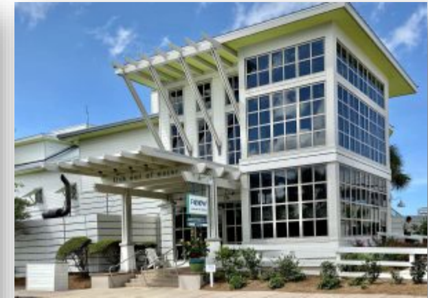
Building Corner or Focal Point
