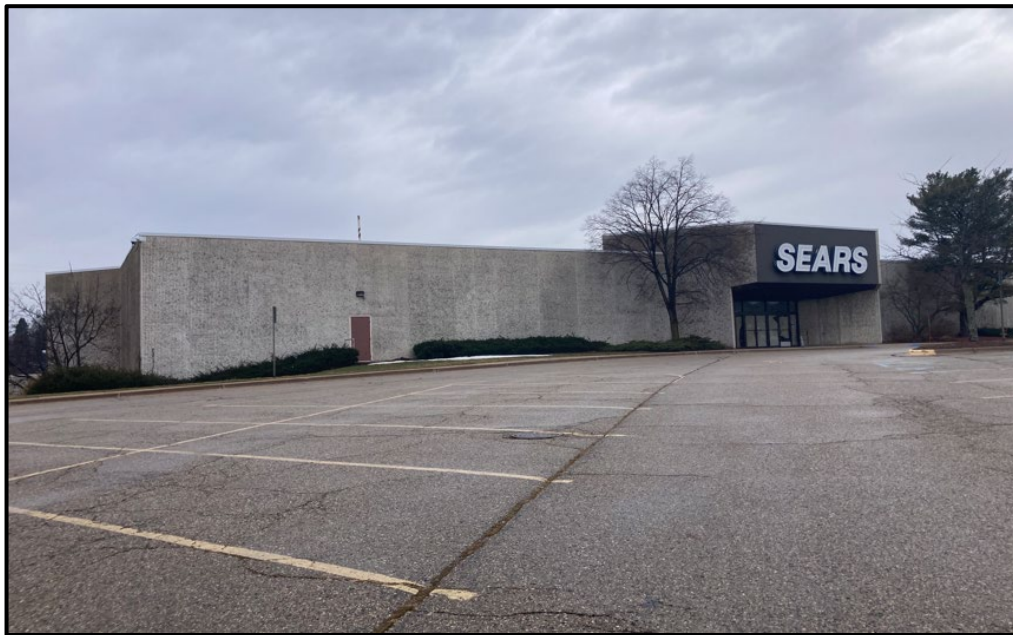
Figure 6: Looking west towards second (upper-level) entrance of the closed Sears.
