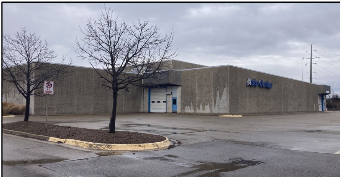
Figure 4: Looking north toward the auto center of the closed Sears tenant within the Crossroads Mall.
