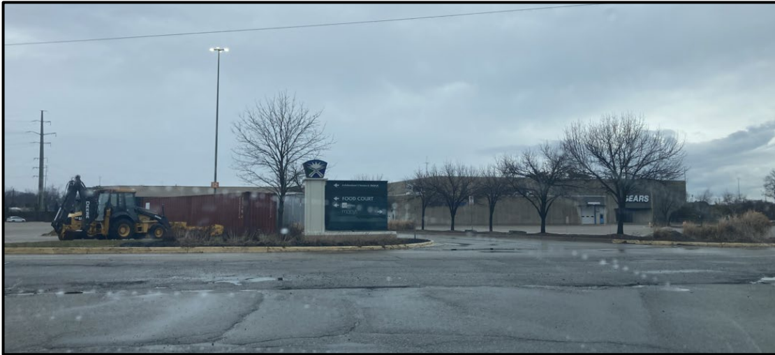
Figure 2: Looking north toward closed Sears tenant within the Crossroads Mall.
